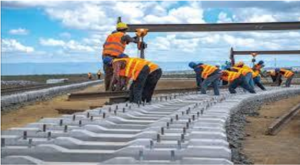
FIGURE 1: LAYING OF THE RAILWAY
